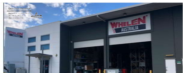
Brisbane, Australia facility
